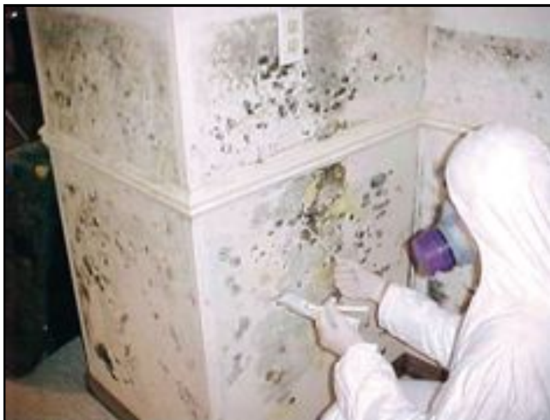
Photo provided by Connie Morbach of Santi-Air Inc. Connie Morbach of Santi-Air Inc. is suited up while testing moldy drywall in a basement after sump pump failure.
